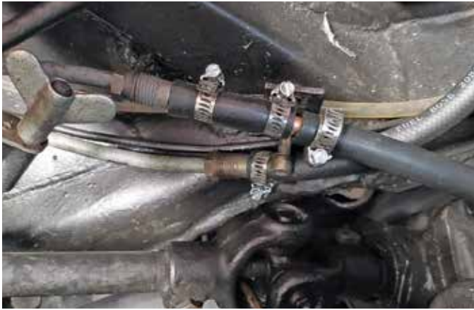
The metal main fuel pipe is connected to the fuel hose that leads to the throttle bodies. The fuel return line from the fuel pressure regulator is connected to the metal reserve fuel line.
