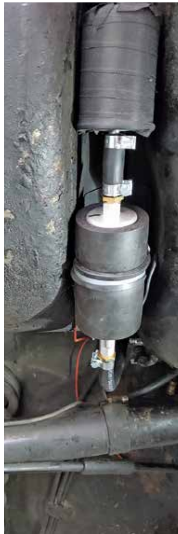
The fuel pump and filter mounted under the trunk between the fuel tank and the second spare tire well.
